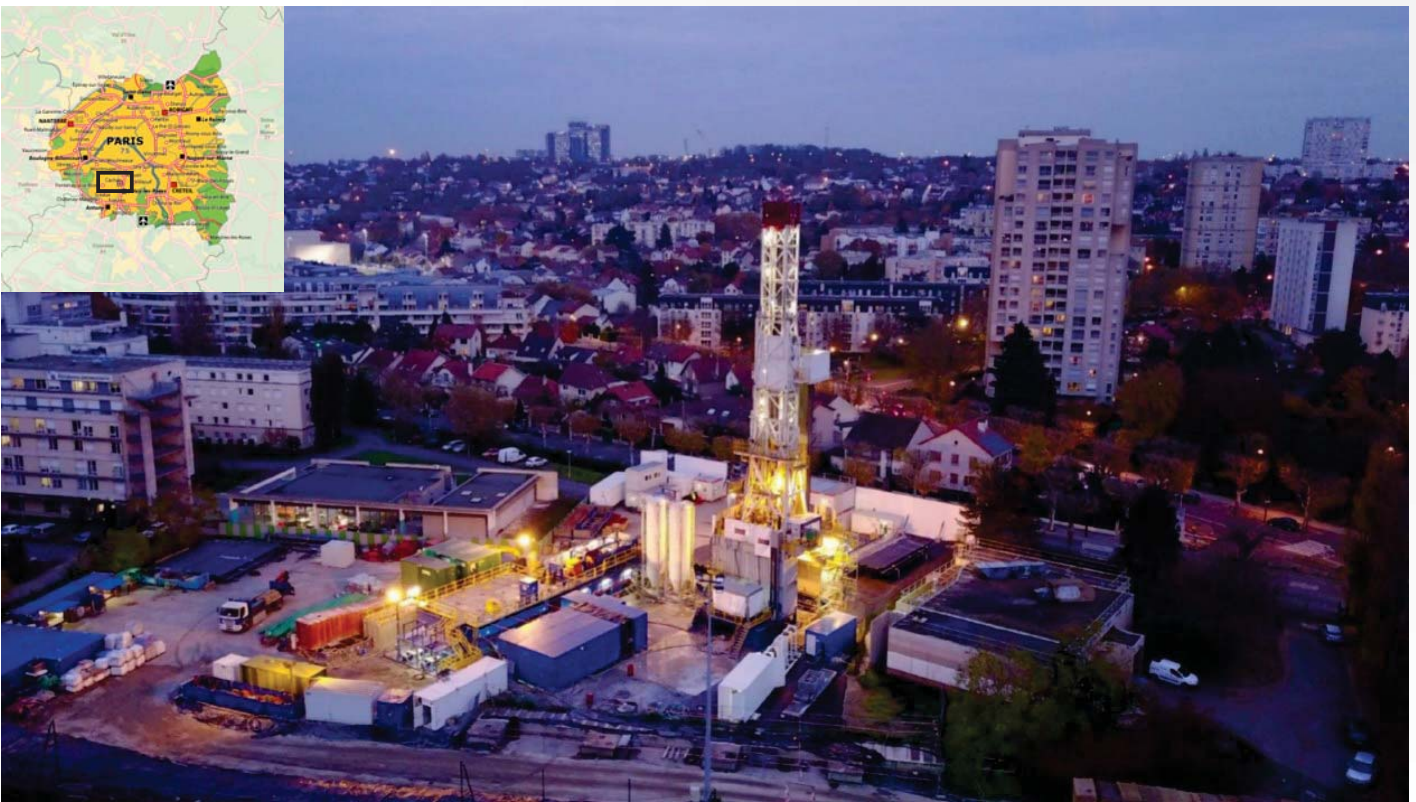
Panoramic view of the Cachan drillsite , 2017
